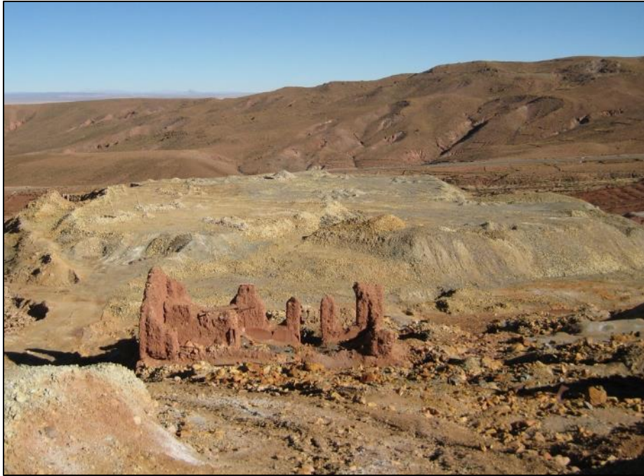
Figure 7.2: View of Pulacayo 1 Tailings/Waste Rock Deposit
